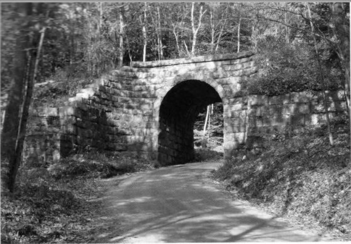
Built in 1848 on the steep hillside above the Ashuelot River's South Branch and just west of the Webb depot area, this granite arch bridge spans Webb Depot Road in Marlborough on a steep, treacherous curve. The arch has an inside diameter of 15.5 feet at the base, a maximum height of twenty-one feet from the crown of the road to the keystone, and a face-to-face width of 30.5 feet. The beautiful curved wings on either side of the arch exemplify the fine craftsmanship used in its mortarless construction. 2012, R. R. Richards Jr. photo.
