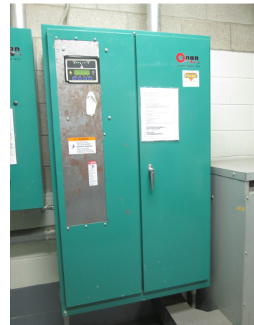
400A Transfer Switch
