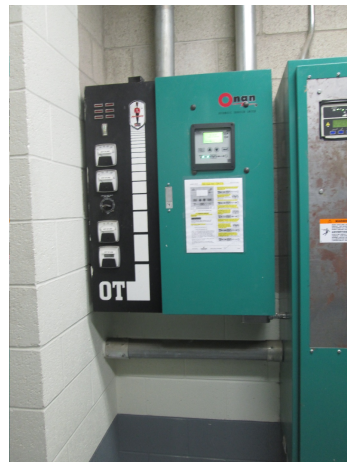
200A Transfer Switch
