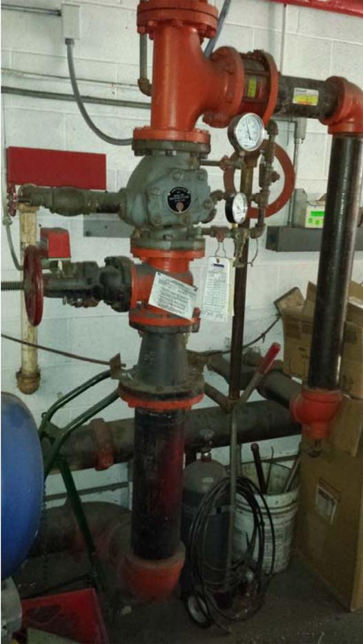
An electrically-driven fire pump located in the boiler room (pictured) boosts system pressure to required levels.
